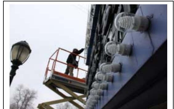
Jeremy Lauffenburger from Denver's Small Business Energy Program replaces old incandescent light bulbs with efficient CFLs on the Bluebird Theater marquee.
